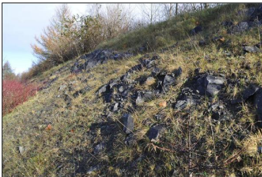
Photo No. 4.1.1 – Existing rock cut on east side of cut between Ch. 130 and 355
